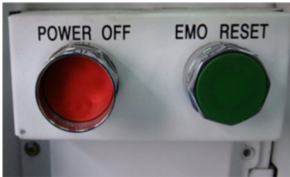
Figure 2-33: PDU power off button for value products
